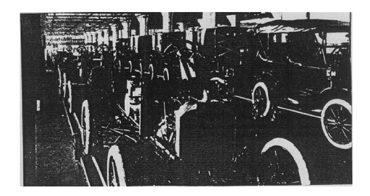
Fig. 1.3 Model Ts Coming off the Final Assembly Line at Ford's Highland Park Plant.
